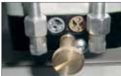
By pass valves and manual release
